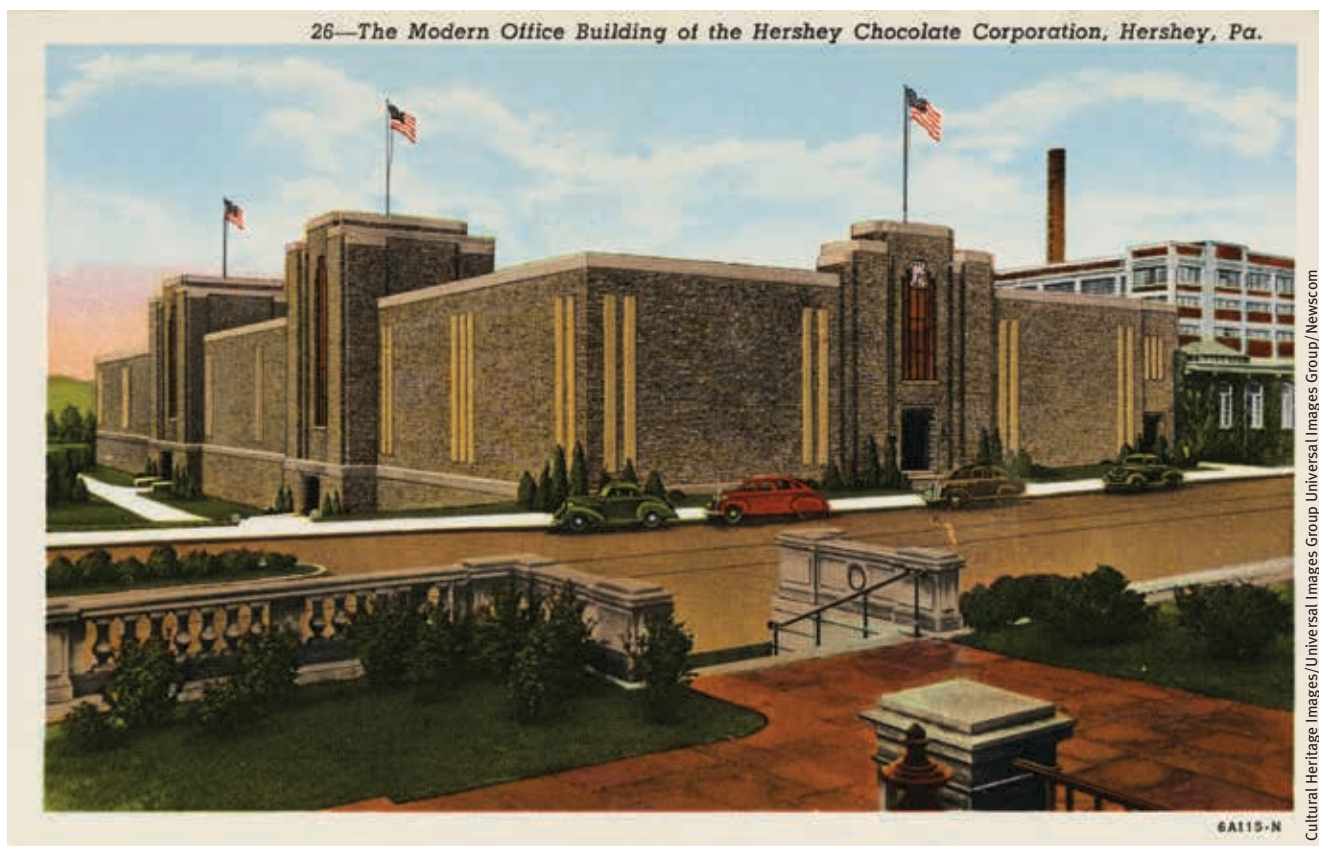
The “modern office building” of the Hershey Chocolate Corp., ca. 1936—windowless, air-conditioned and indirectly lighted.
