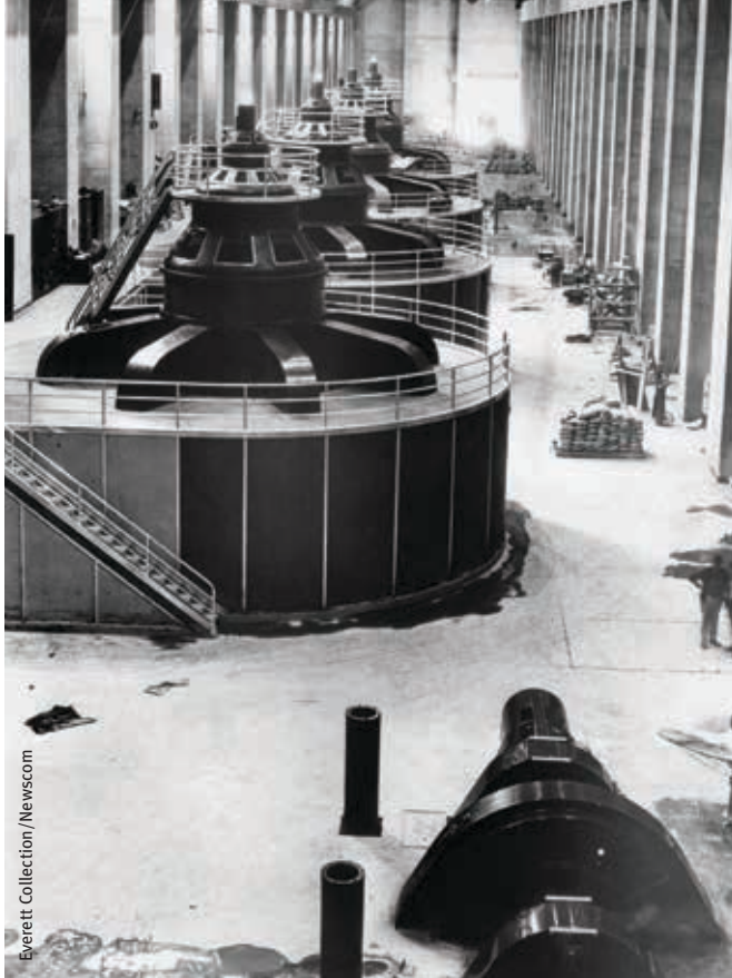
Generators at the Hoover Dam power house, 1937.
