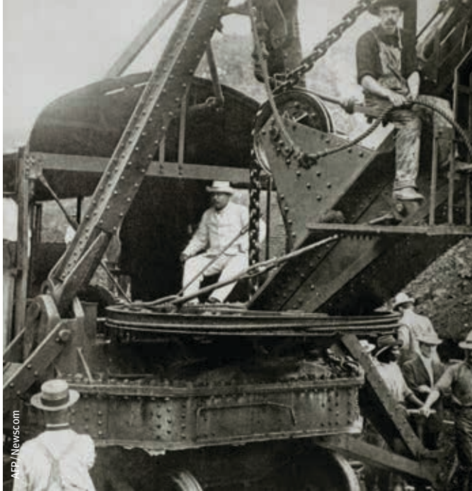
This November 1906 file photo shows President Theodore Roosevelt (center) sitting on a steam shovel at the Culebra Cut of the Panama Canal.
